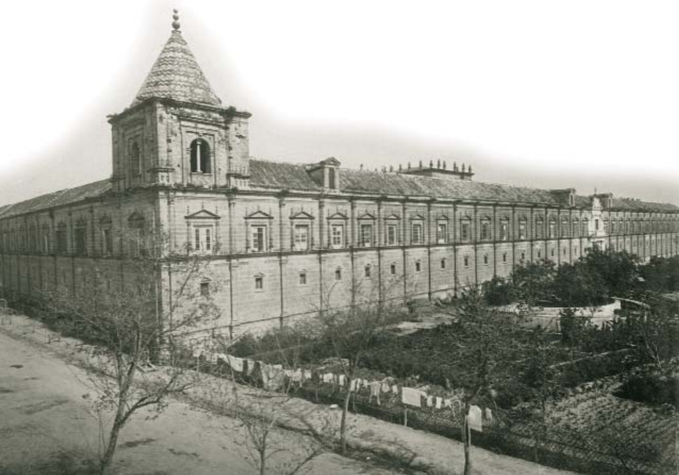
Seville, c. 1870. General view of the Hospital de la Sangre.
