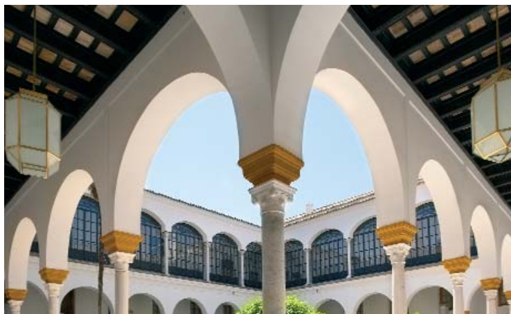
Intersection of two galleries in the Patio del Alcohol.
