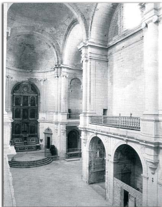
Church interior during restoration.
