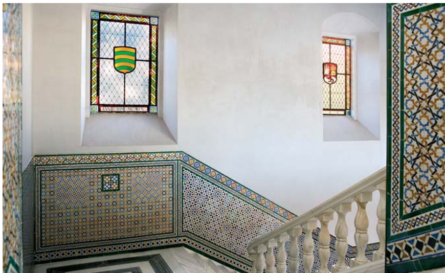
Patio del Cardenal stairway after restoration.
