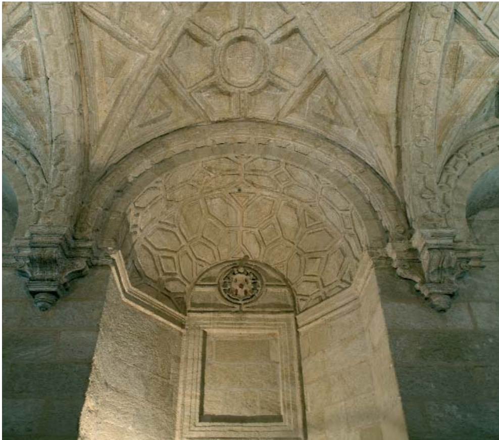
Church sacristy vault.
