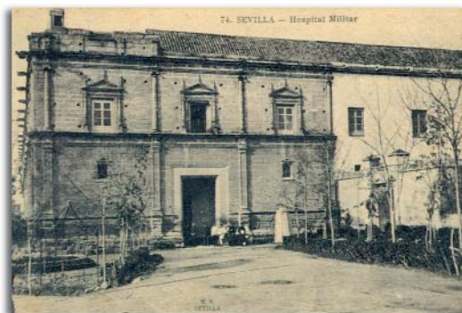
Photograph of one of the building's doors.
