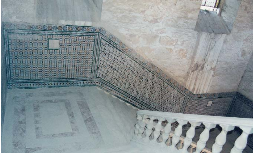
Patio del Cardenal stairway before restoration.
